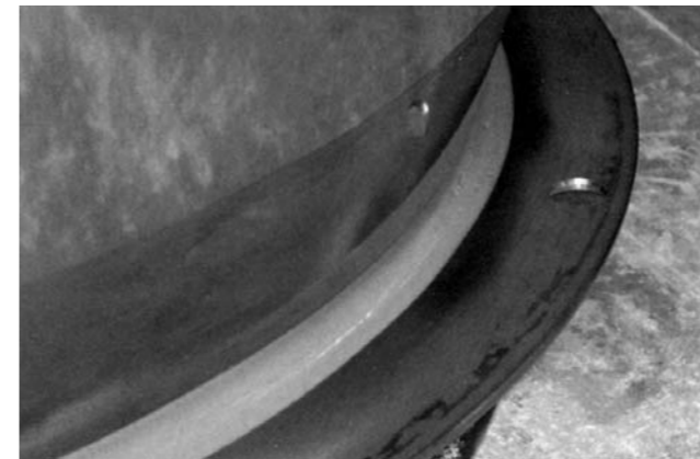
Fig. 11: External crevice at base of hopper sealed with FDA approved epoxy
