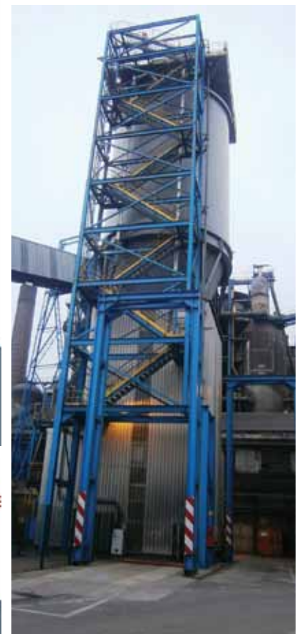
Photo of the completed installation
