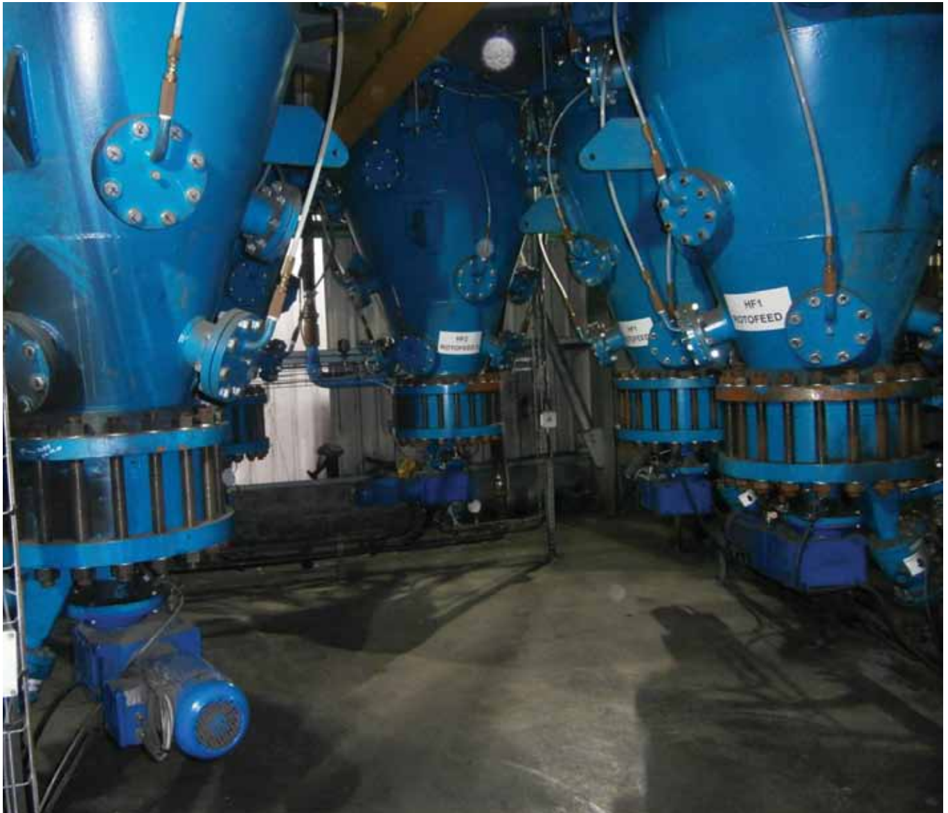
Photo of the tandem Rotofeeder under the silo
