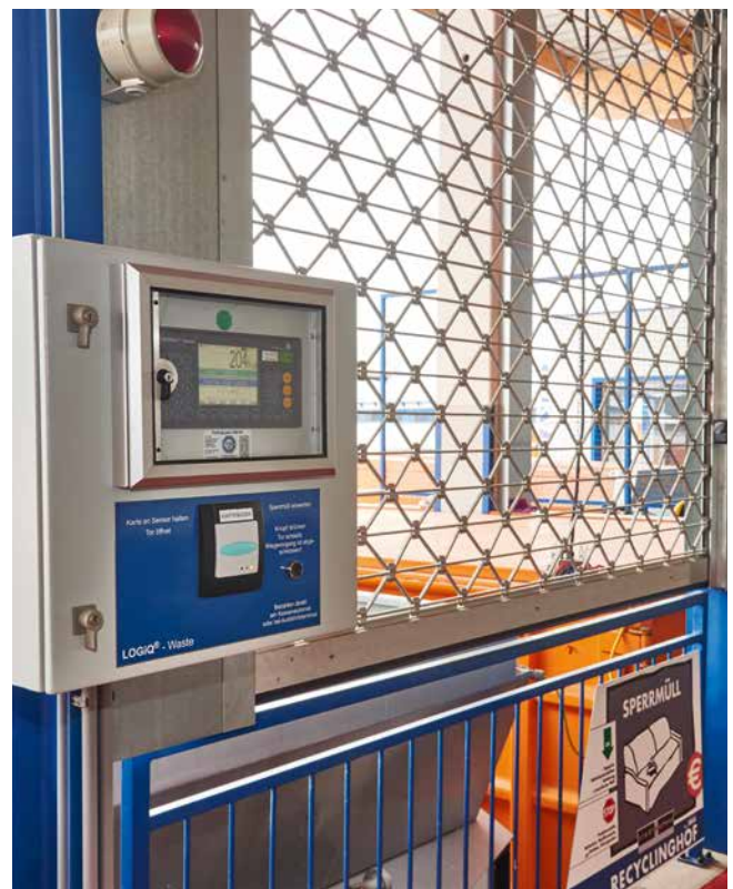
Photo 5: At the disposal stations, waste is weighed in 1 kg loads.
