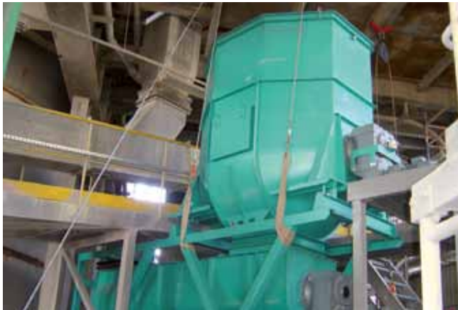
Figure 6: MultiFlex screw weighfeeder when lifting into plant.
