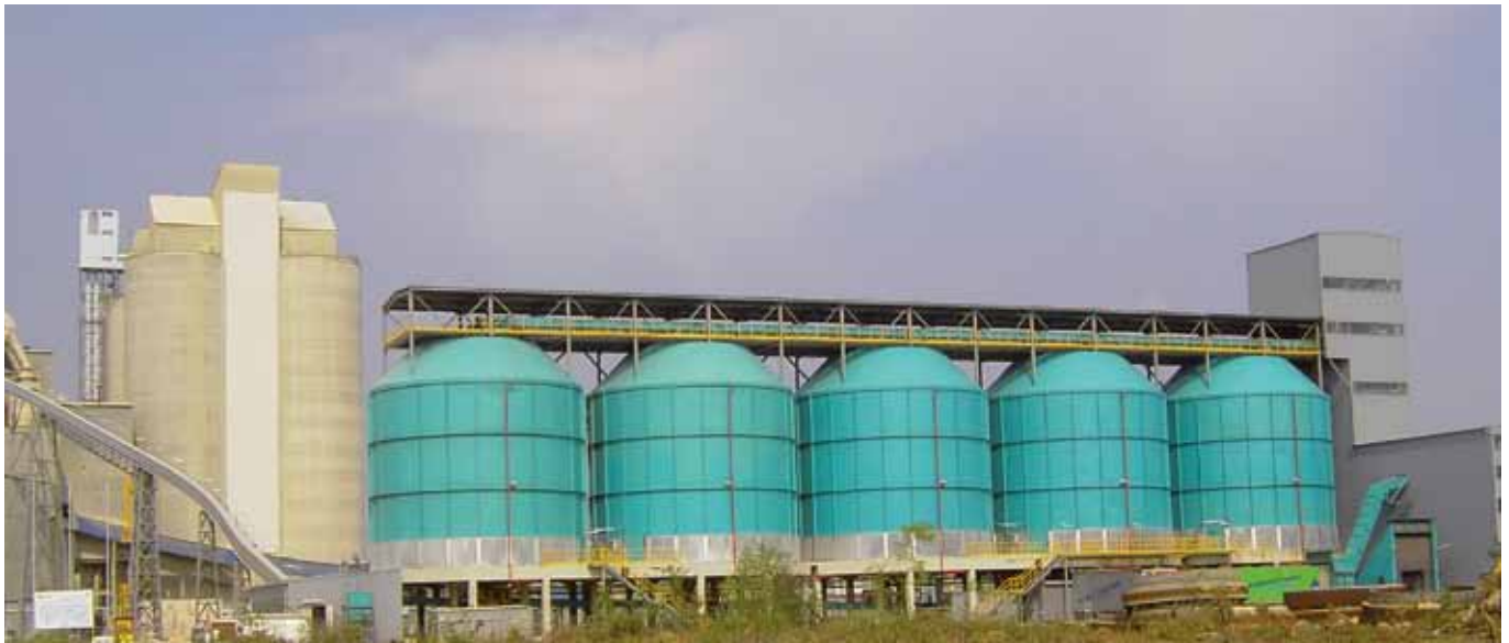
Figure 2: Alternative fuels installation at Ożarów
